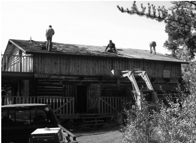
The Naturelore building gets a new metal roof with skylights.
